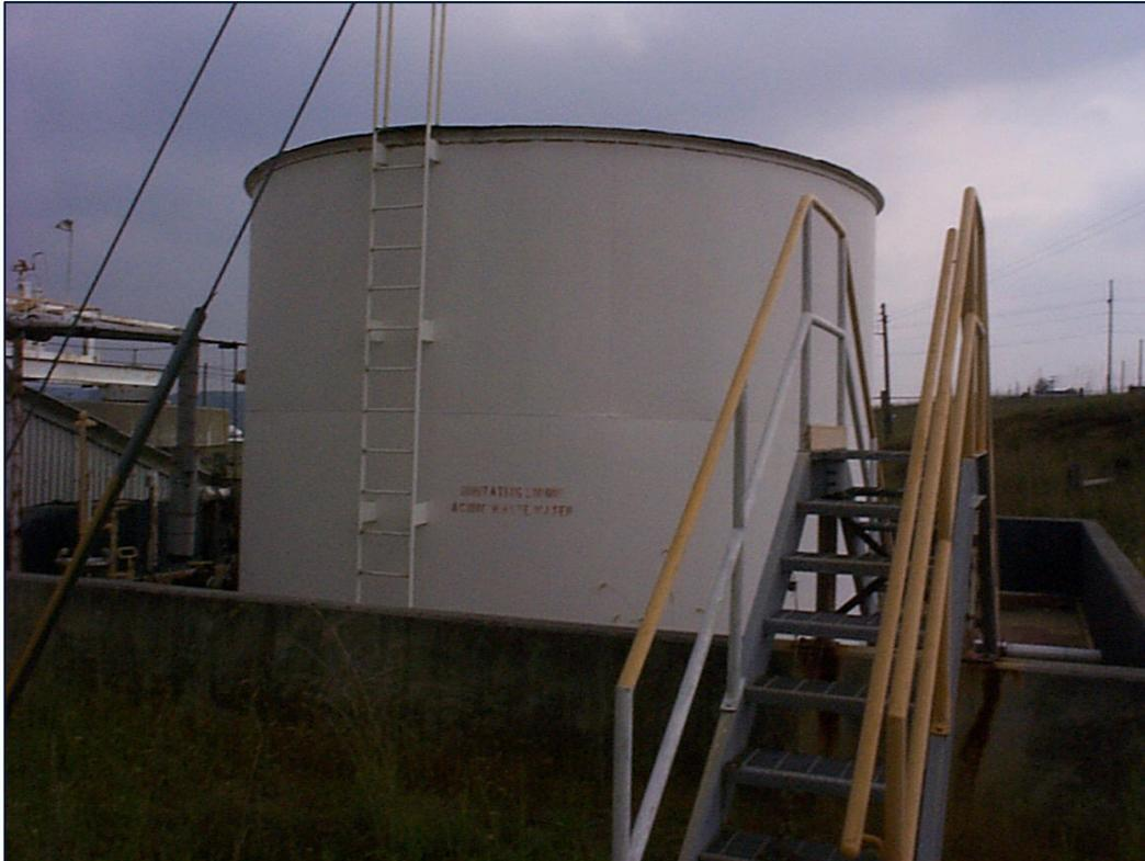
**PHOTO 6: SSA 18 – Unit 18f Steel Wastewater Surge Tank**
