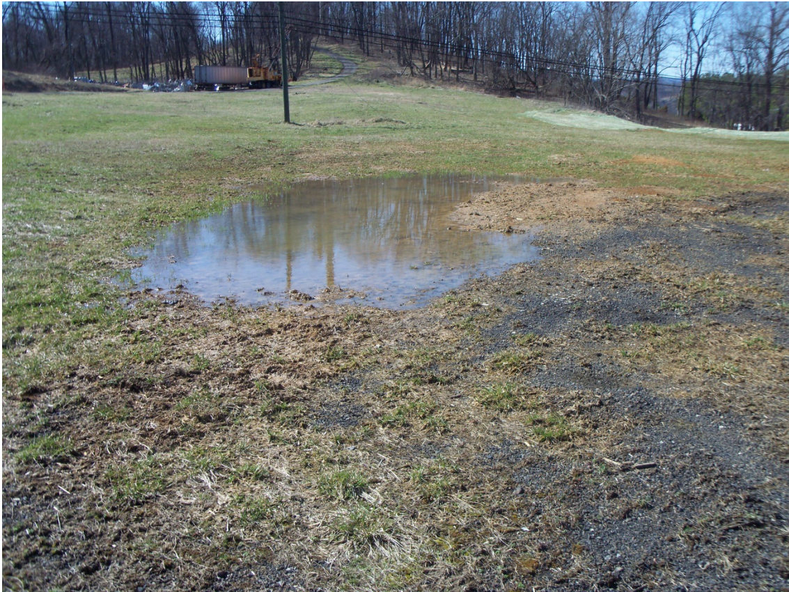
Photo 5 – Areas of ponding noted during second Quarter of LTM-3-2012.
