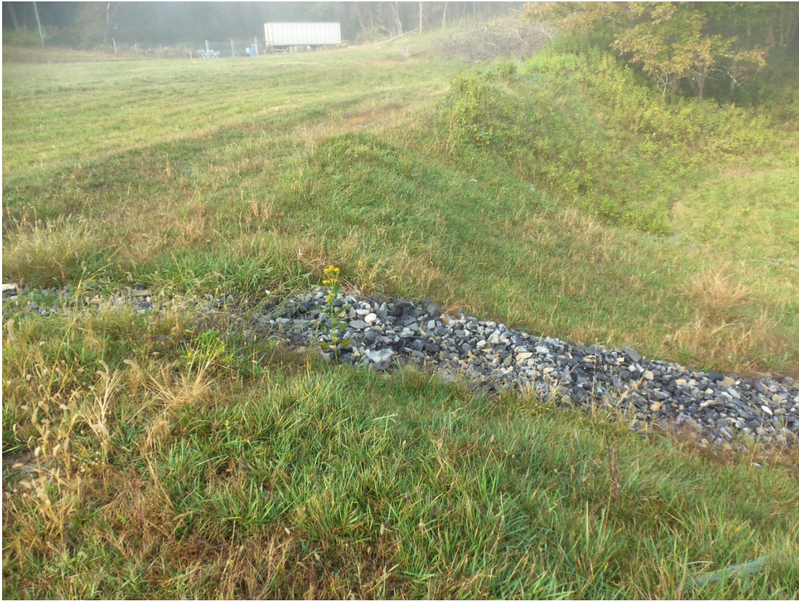
Photo 13 - SWMU 40 drainage swale view during Quarter 4 inspection, 9-2012.
