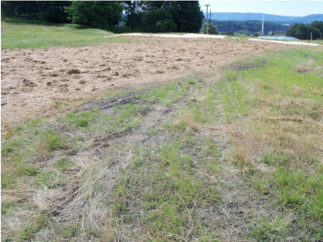
Photo 9 - SWMU 40 final grade with seed and straw after drainage improvement-Quarter 3, 6-2012.
